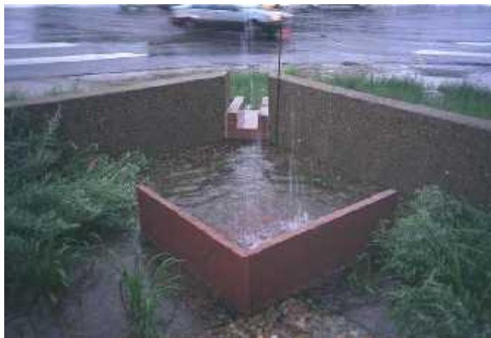
Front holding pond Plants will be watered by runoff from the roof
