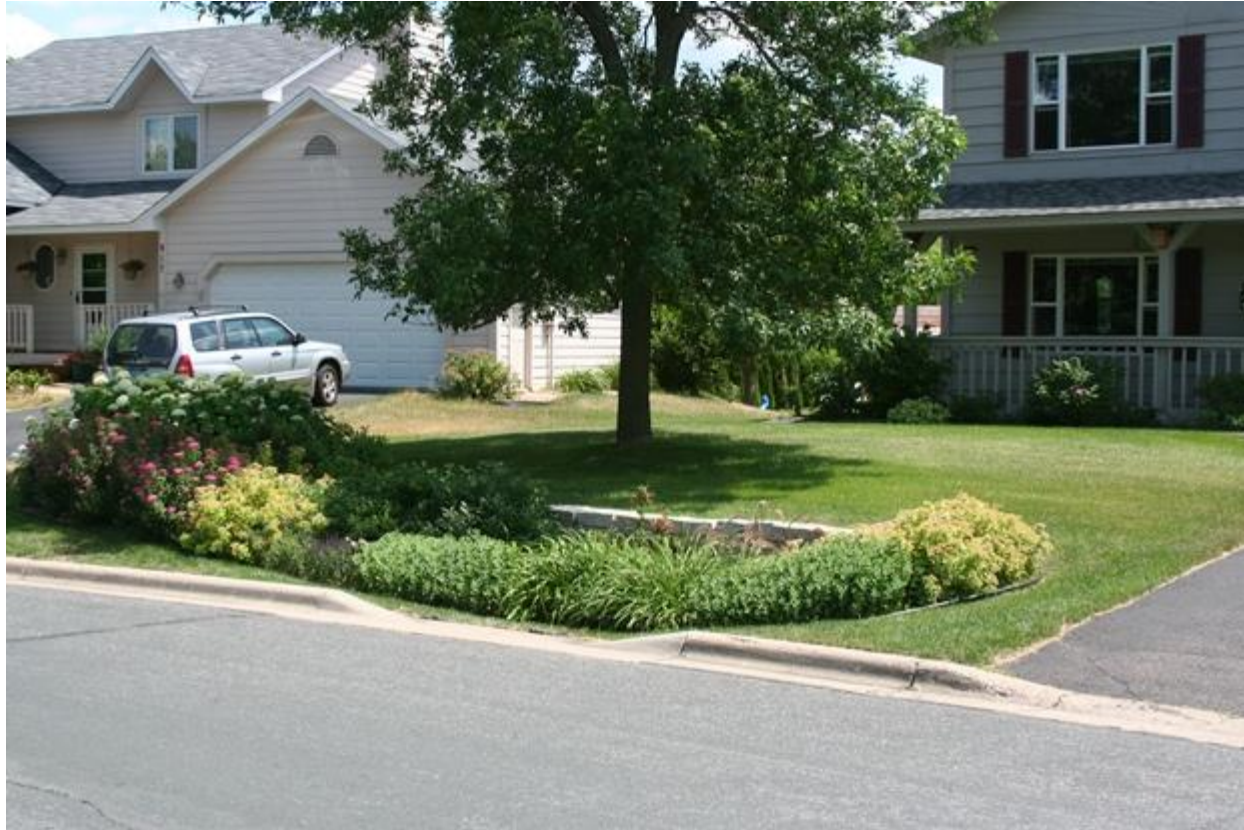
Figure 1: Bioretention cell in residential area. Note curb-cut where stormwater enters from street. (Photo: LeFevre)
